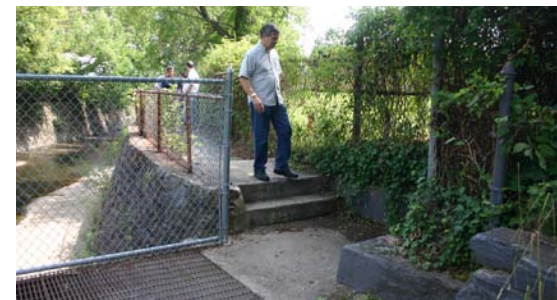
Photographs (counter clockwise): Segment #5, PECO Right-Of-Way south of Garrett Road; Segment #5B, Catwalk on bridge abutment; and access to Beverly Boulevard.
