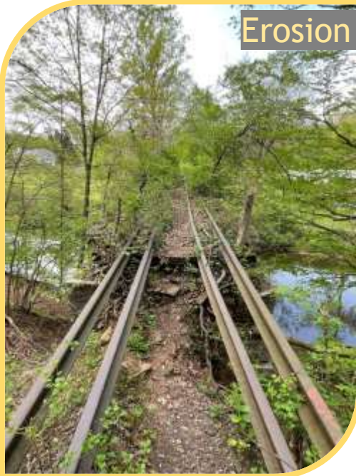
Failed Drainage Features
