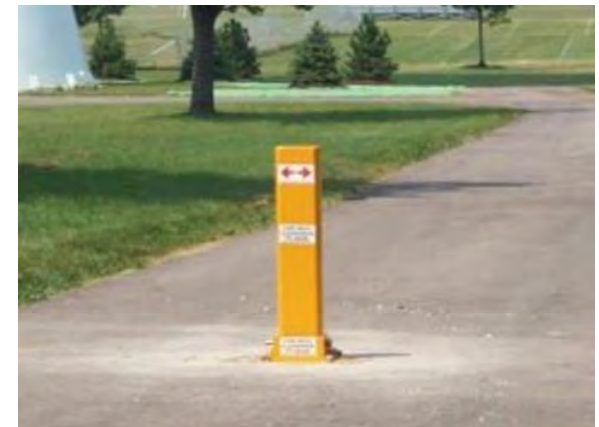
Bottom: Removable or collapsible bollards can restrict vehicles while still allowing access for emergency and maintenance vehicles.
